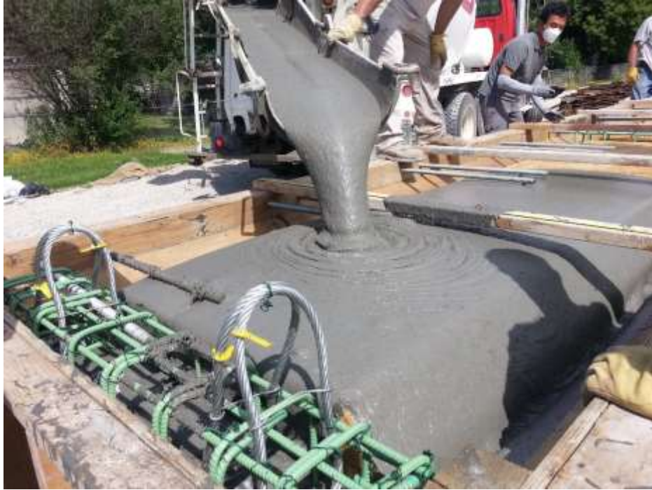
Figure 5-18 K-UHPC Pouring for Sixth Girder
