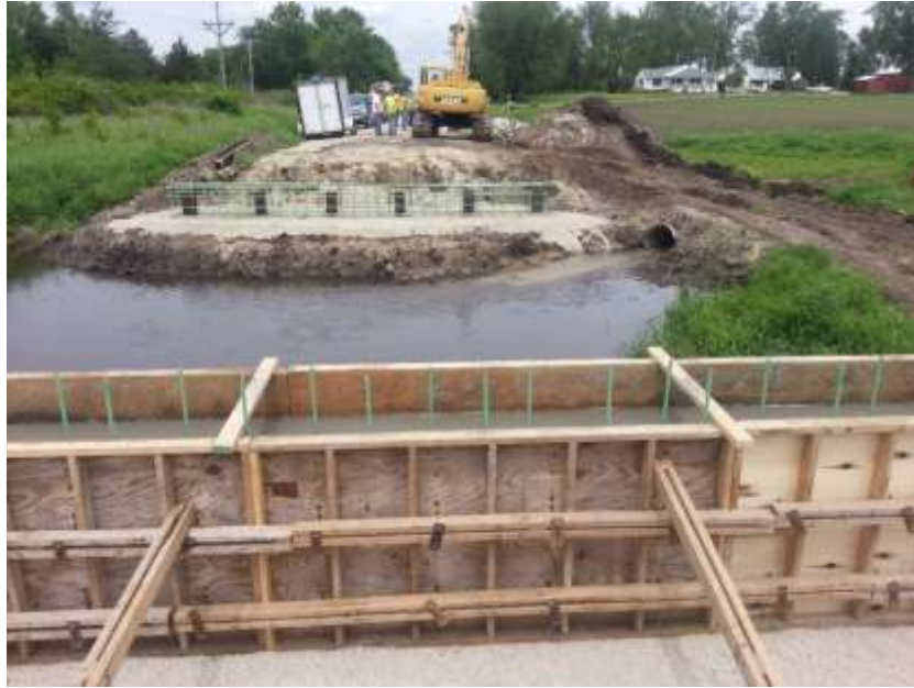
Figure 4-2 Construction of Substructure of Hawkeye UHPC Bridge
