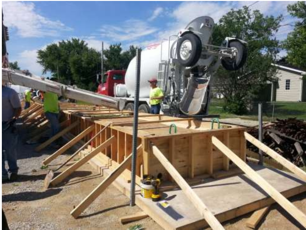
Figure 5-2 Orientation of Two Trucks during Pouring
