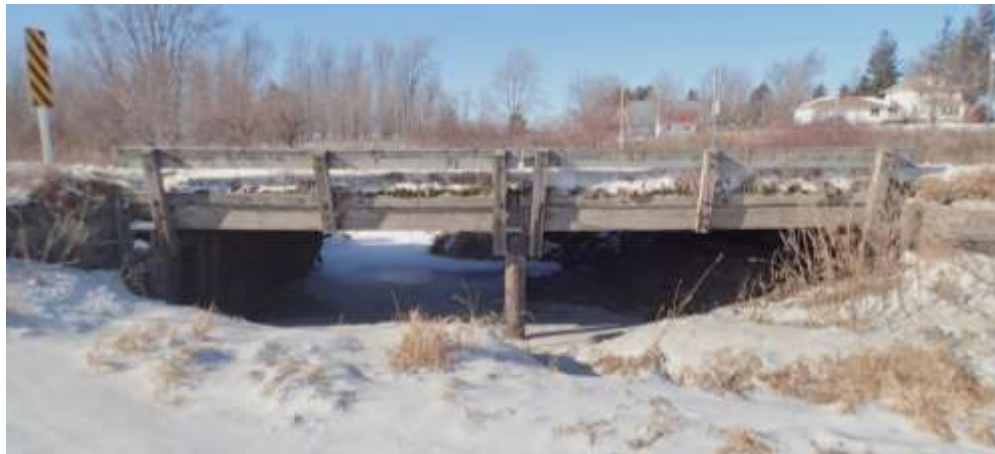
Figure 2-4 Old Multi-Beam Timber Bridge
