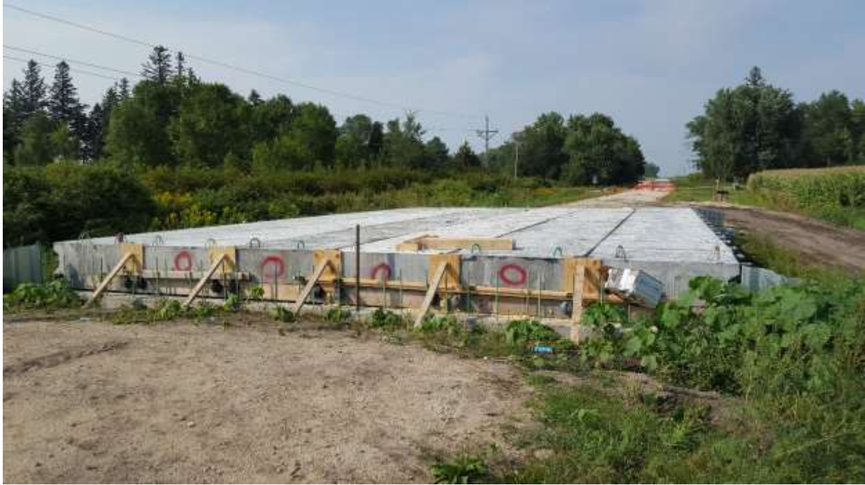
Figure 5-33 Formwork for Joint Filling
