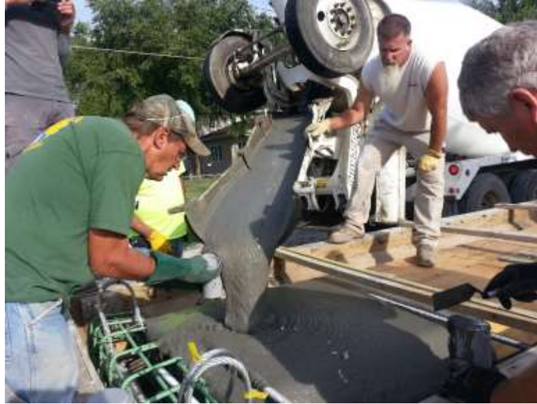
Figure 5-17 K-UHPC Pouring for Fifth Girder
