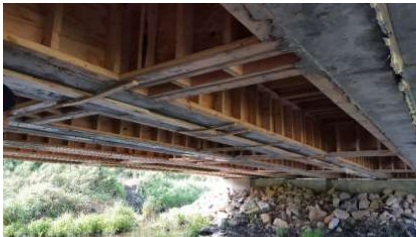
Figure 5-32 View from Under the Bridge
