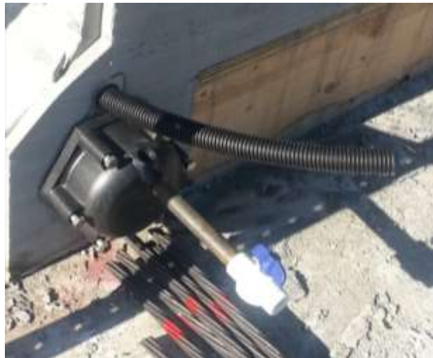
Figure 5-22 Cap with Attached Grout Opening
