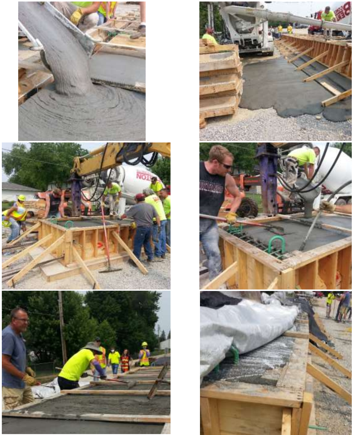
Figure 5-11 Second Girder Construction
