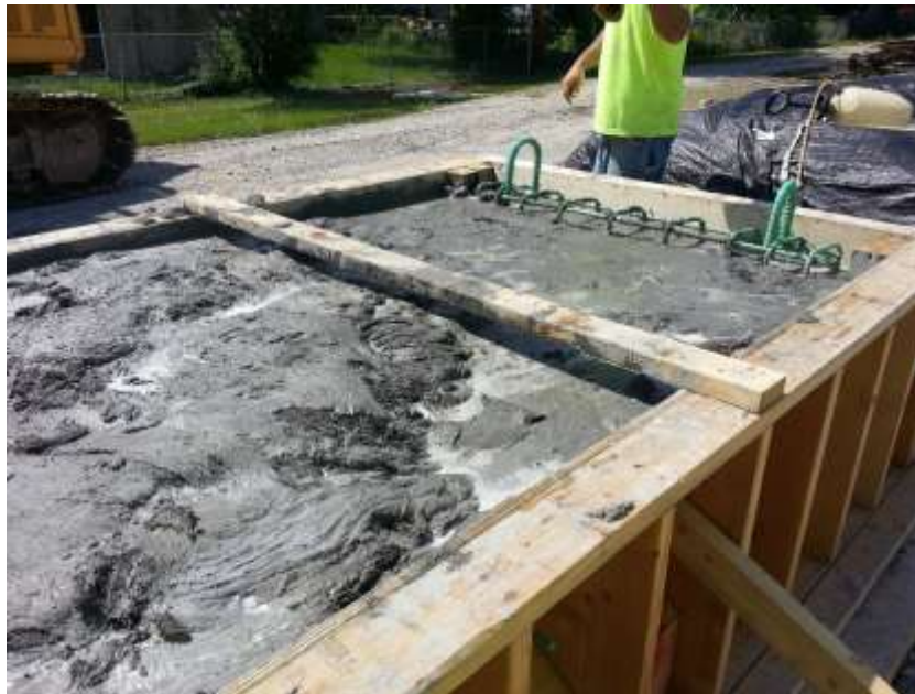
Figure 5-5 Incomplete Second Girder
