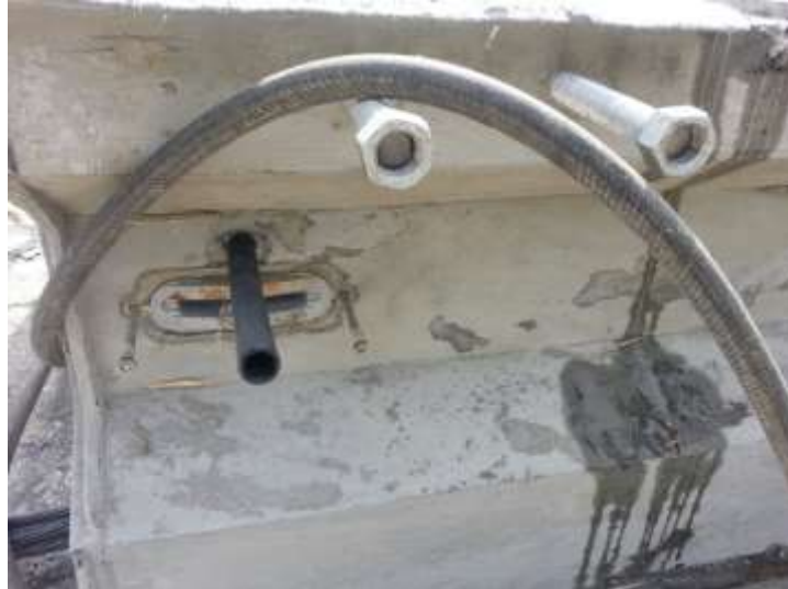
Figure 5-20 Opening for Transverse Post-tensioning Strands
