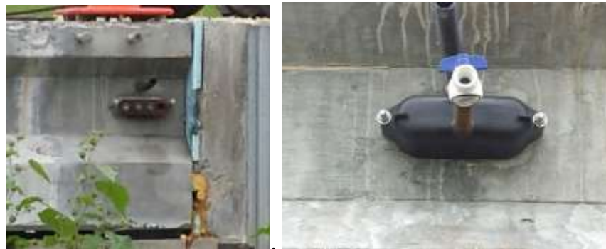
Figure 5-40 Post Tensioned Transverse Strands with/without Cap
