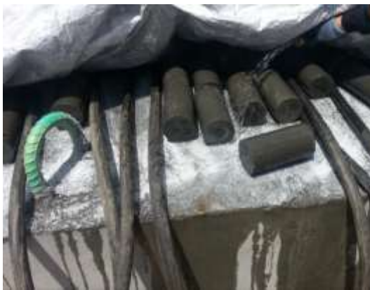
Figure 5-7 Steam Curing of First Girder
