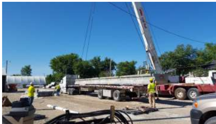
Figure 5-26 Girder Delivered onto a Truck
