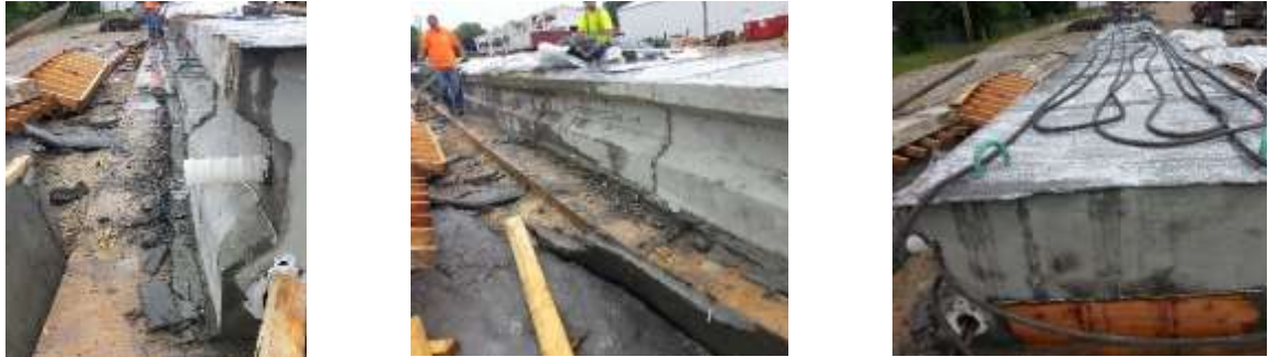
Figure 5-12 Completed Second Girder
