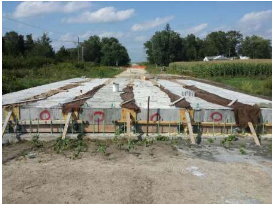
Figure 5-36 Burlaps Put on Each Joint
