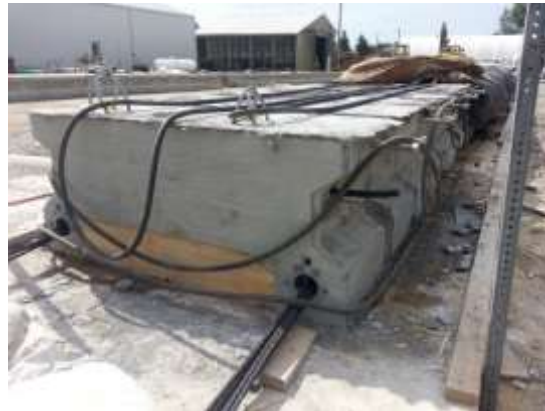
Figure 5-19 Steam Curing on Sixth Girder
