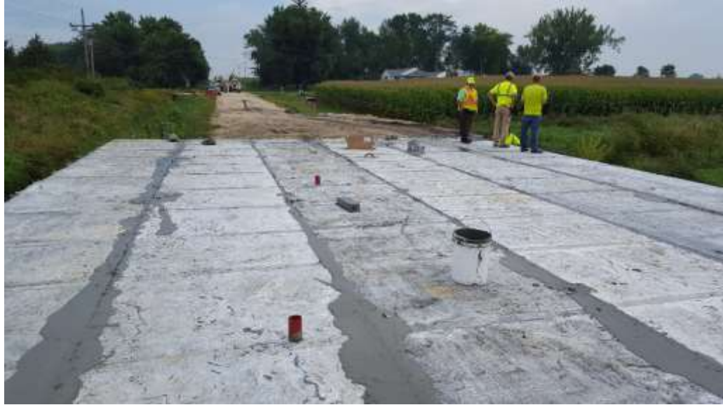
Figure 5-35 Filled Joints with K-UHPC
