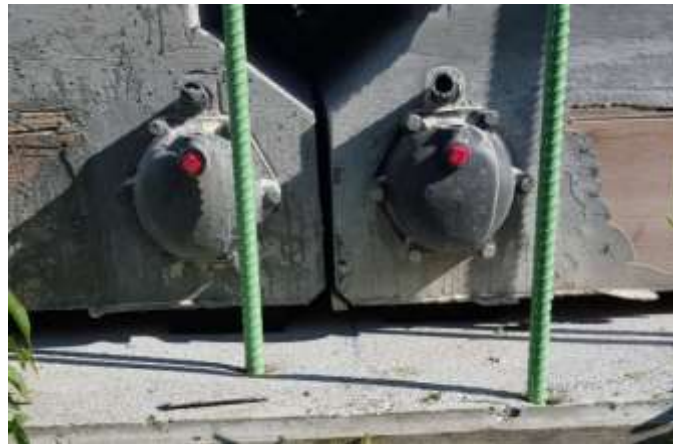
Figure 5-29 Steel Plates between Abutment and Girders
