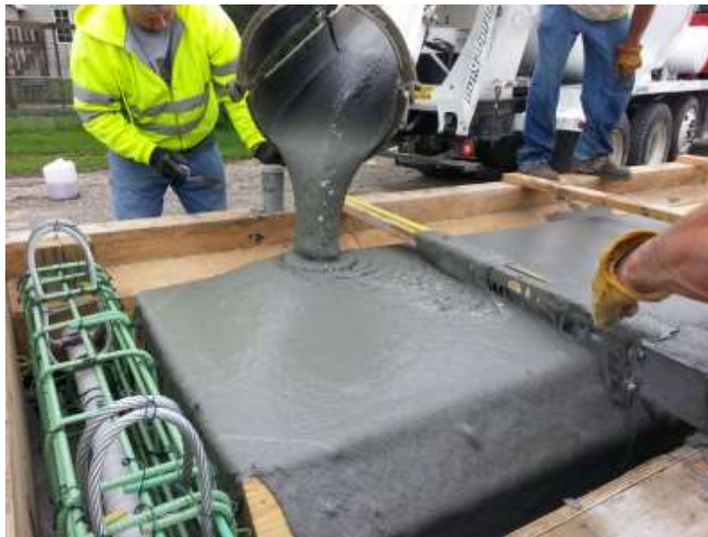
Figure 5-15 K-UHPC Pouring for Third Girder
