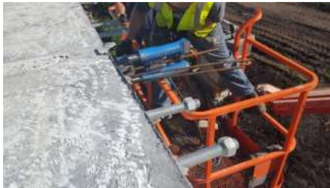
Figure 5-37 Transverse Post-tensioning
