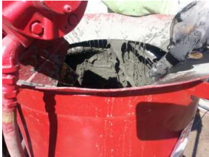
Figure 5-23 Grout in a Mixer
