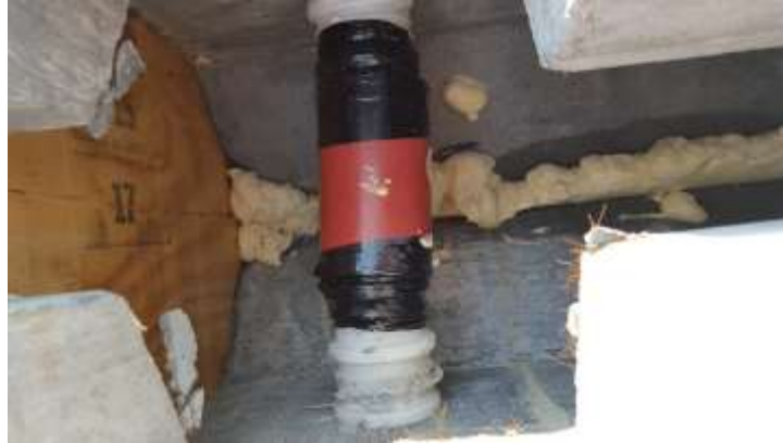
Figure 5-31 Filled Gap and Connected Post-tensioning Duct
