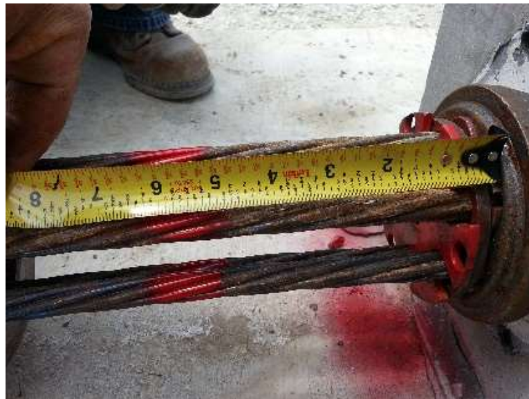
Figure 5-14 Elongation of Post-tensioned Strands
