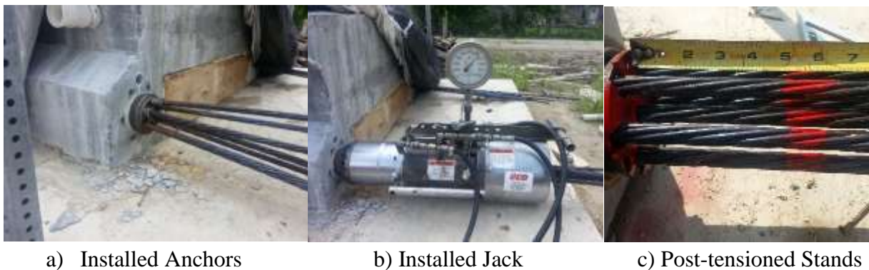
Figure 5-10 Post-tensioning on First Girder
