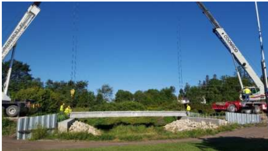
Figure 5-27 Bridge Installation
