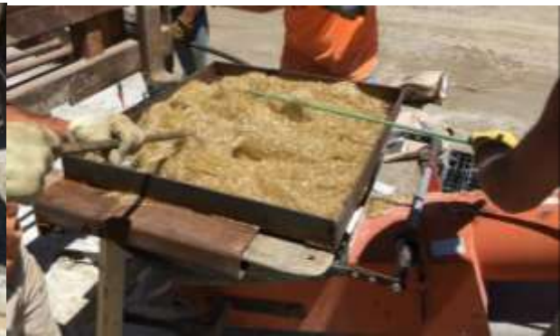
Figure 5-1 Adding K-UHPC Constituents
